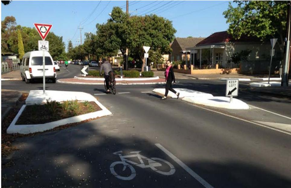
**Figure 7. Tangential roundabout redesigned to radial, Beulah Road, Norwood, SA (source: GTA Consultants)**
